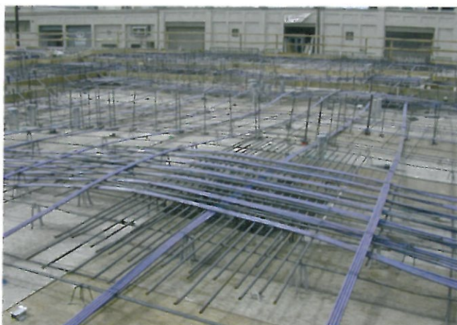
(a) Minimum of two tendons over support (P423)
