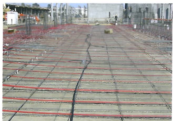
(b) Distributed tendons placed parallel (P424)
