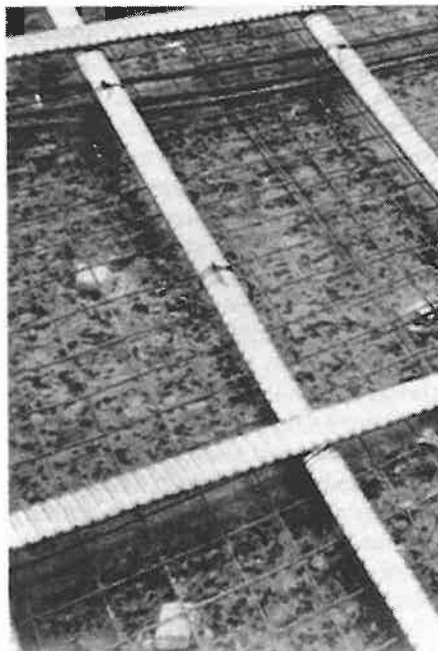
Fig. 4 — Slab reinforced with bonded tendons.
