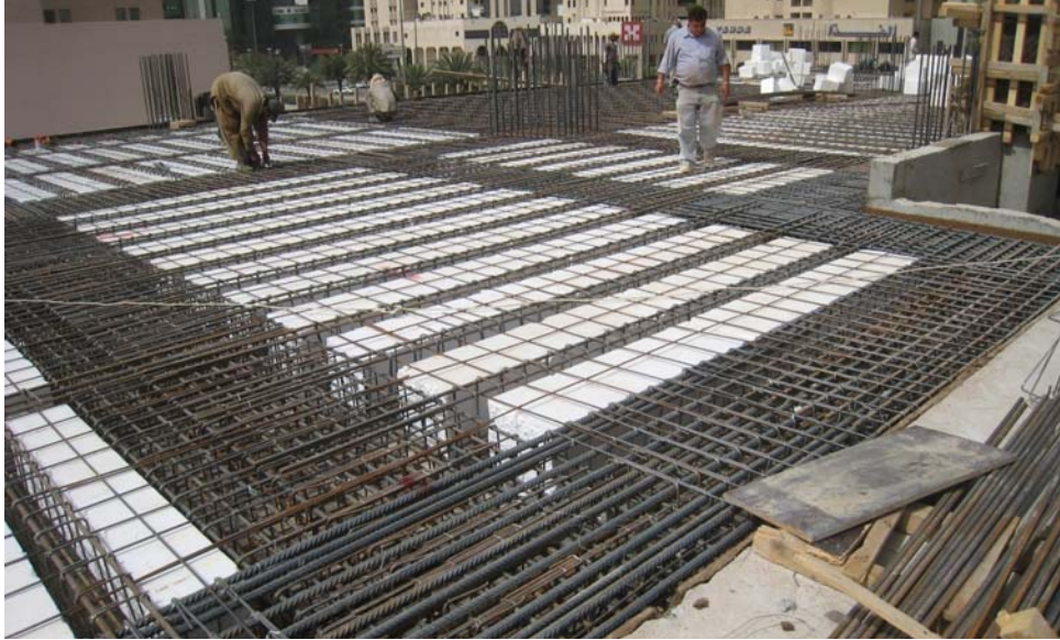
FIGURE 1-3 Application of Styrofoam Blocks to Create Voids in a Slab
