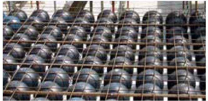
(b) View of a voided slab in construction
