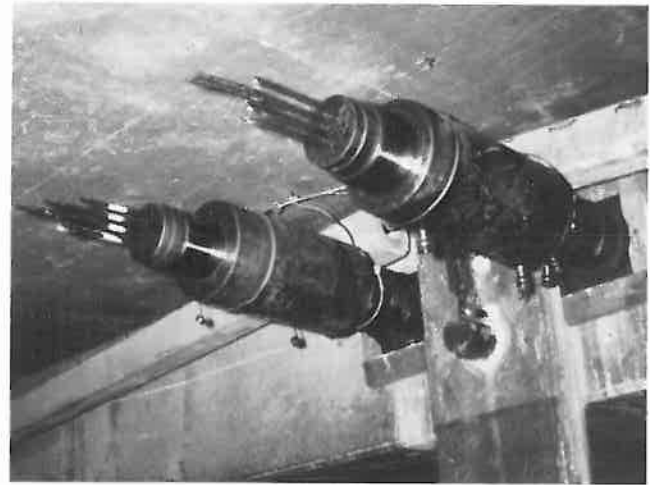
Fig. 10 — Transfer girders were stressed from within the parking garage.
