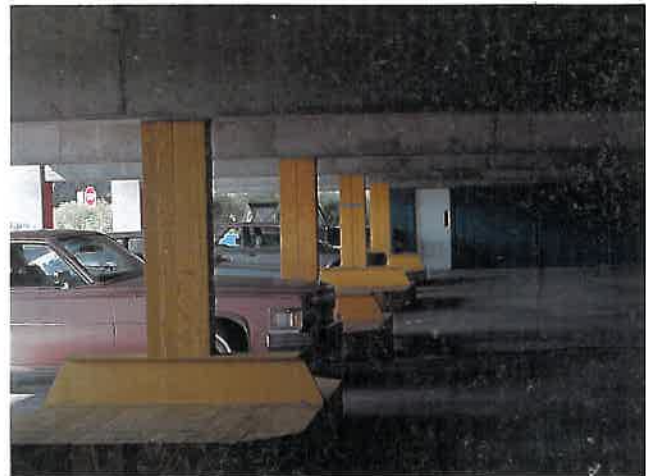
Fig. 2 — (below, right) Prior to rehabilitation, deterioration of the structure had necessitated extensive shoring.
